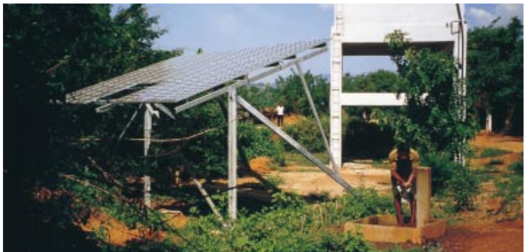
A solar-powered electricity generator of the type to be installed in the Philippines.
